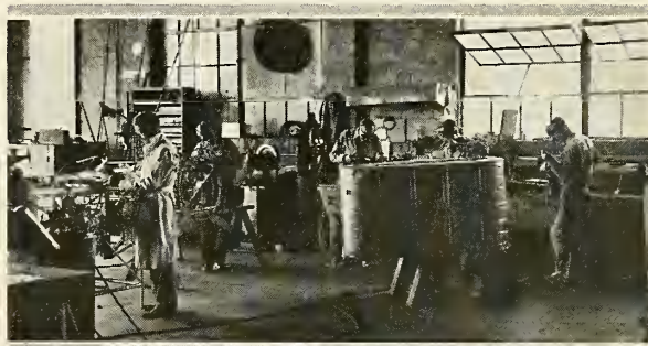
Constructing the 180-gallon fuel tank for a Fokker trimotor
